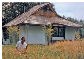
Builders of the Pacific Coast page 38 Stefan Doll's House, built by Lloyd House, British Columbia, Canada
