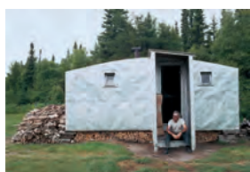
Home Work: Handbuilt Shelter page 151 Frank's home (made by him of local spruce and sheet metal for $35), Nova Scotia, Canada
