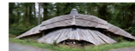
Builders of the Pacific Coast page 99 Woodshed by Peter Buckland at Cougar Annie's, British Columbia, Canada
